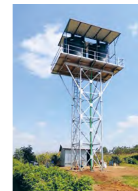
The new water tower in Mbakalo ward.
