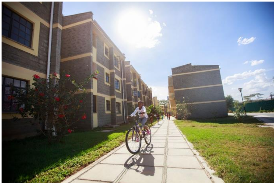
Pedestrian walkway at Riverview. Wide walkways increase pedestrian safety.
