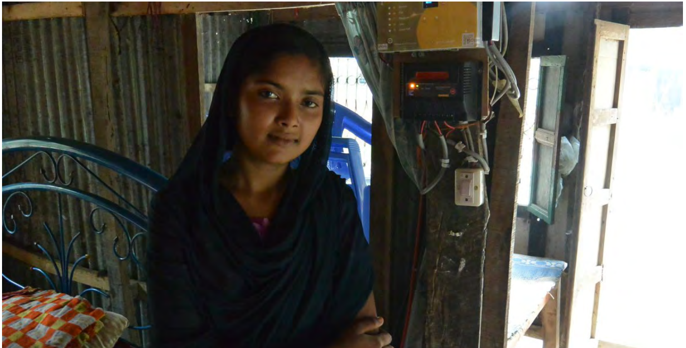
A resident stands next to a SOLbox, which electrifies her home and village in rural Bangladesh.
