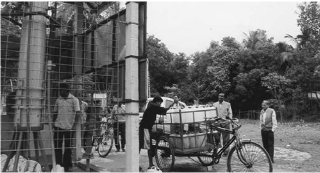
A Drinkwell water facility in West Bengal.
